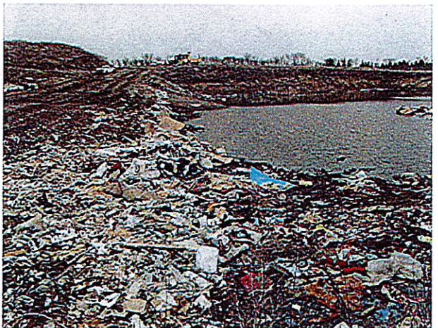
View from south-central portion of burial area, facing north
