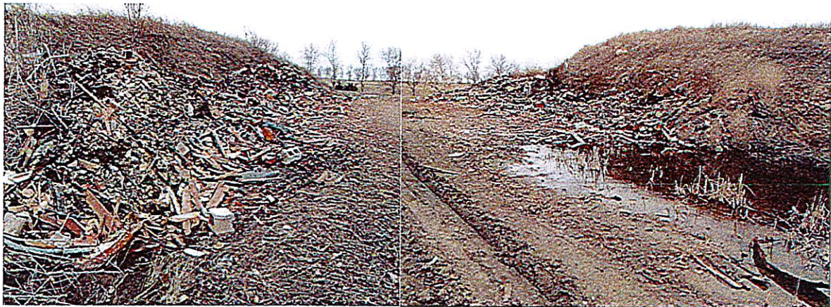
Burnt demolition debris, facing north NW corner of site
